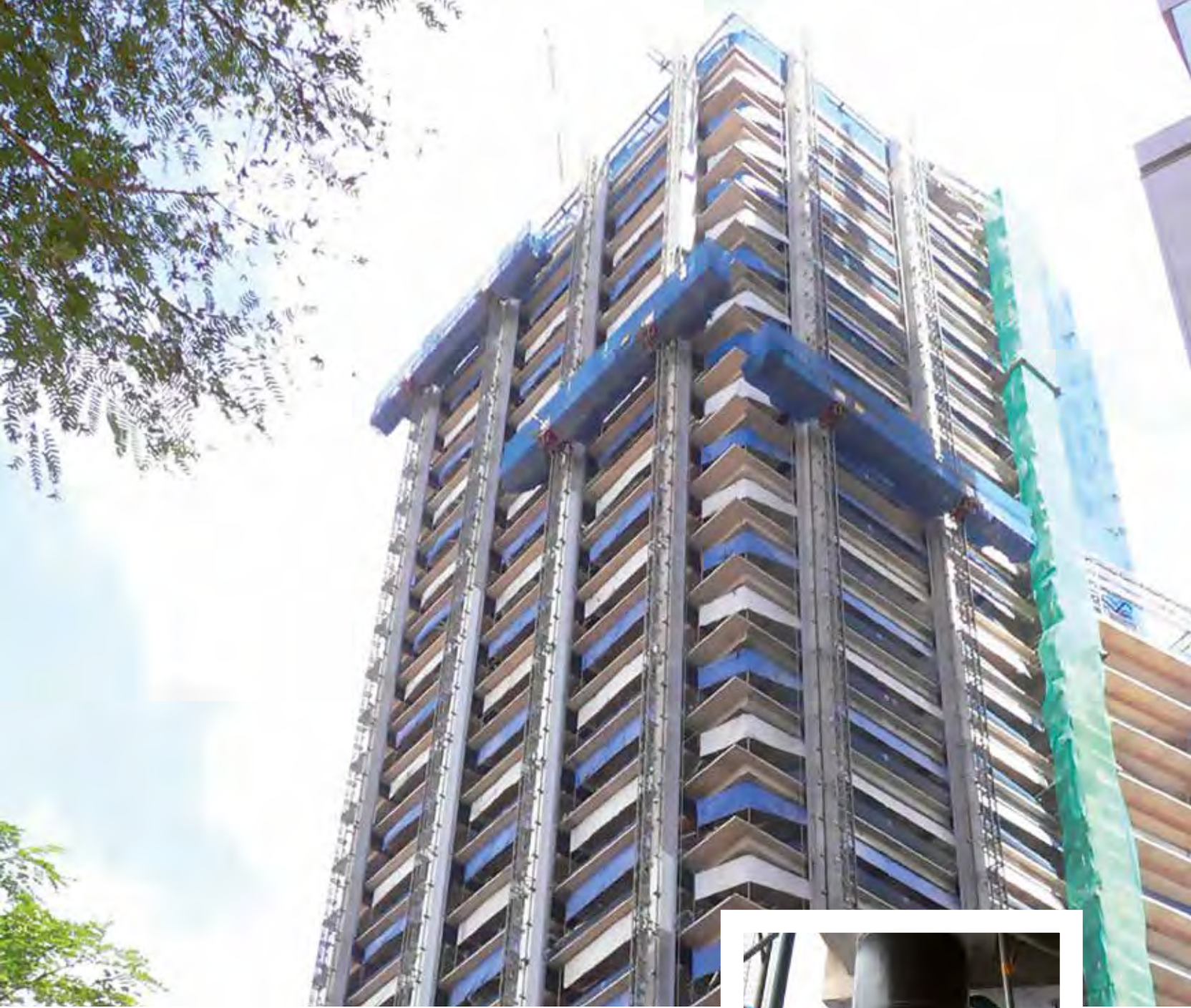
↓ HOUSING & DEVELOPMENT BOARD Singapore | 2013
